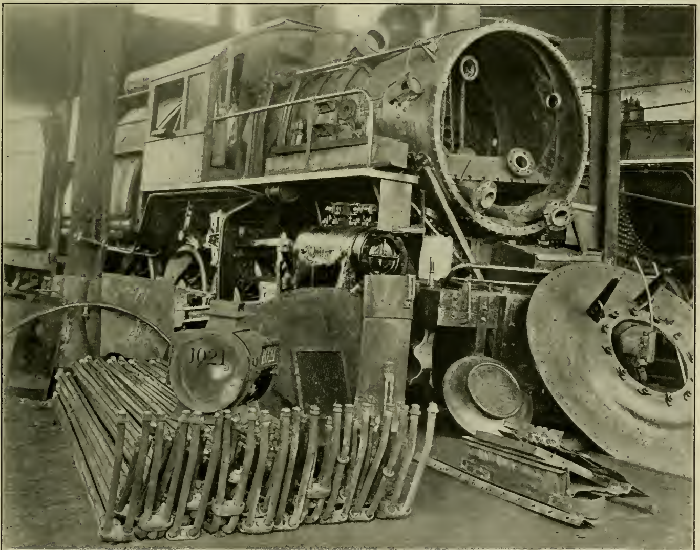
Engine as Dismantled to Regrind Dry Pipe Connection
